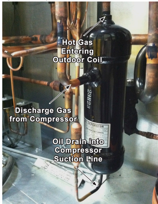
Figure 22: Oil Separator
