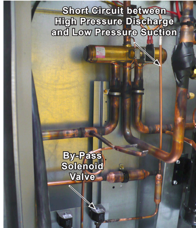
Figure 28: By-pass Solenoid Valve
