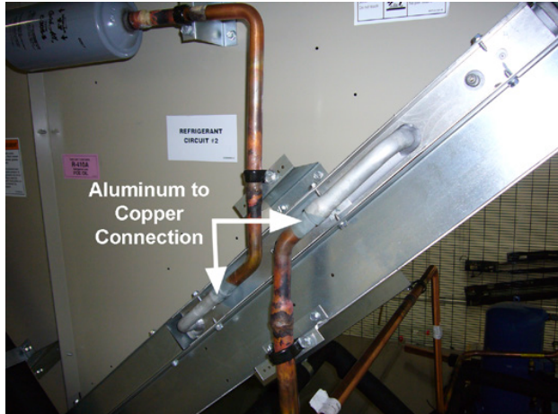
Figure 83: Aluminum/Copper Connection
