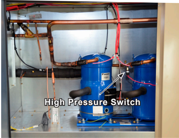
Figure 33: High Pressure Switch
