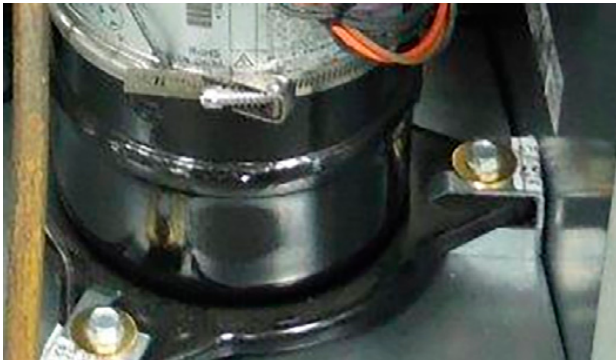
Figure 18: Compressor Brackets
