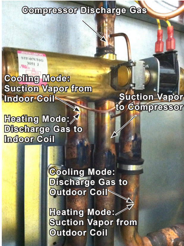
Figure 27: Four-Way Valve
