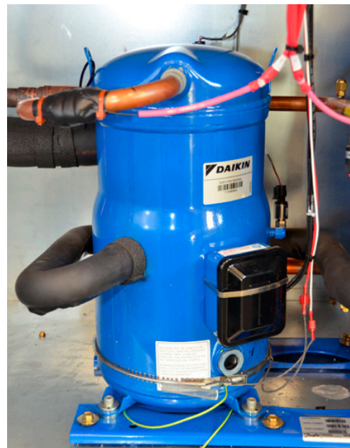
Figure 32: Compressor Suction and Discharge on DPS 025–028 units
