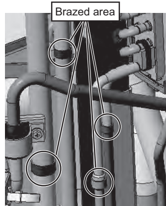
Removal of the right rear heat exchanger on a standard model (Figure 16)
