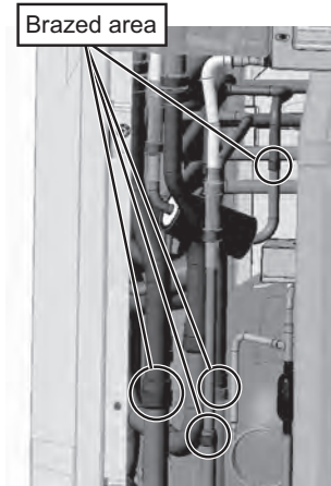
Removal of the front heat exchanger on a high-efficiency model (Figure 11)
